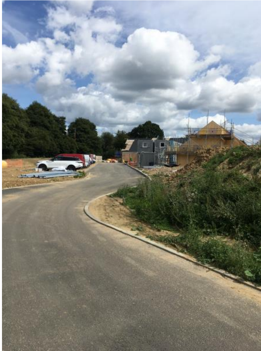
Photo 5 : View of part of Block D and Block C facing east
