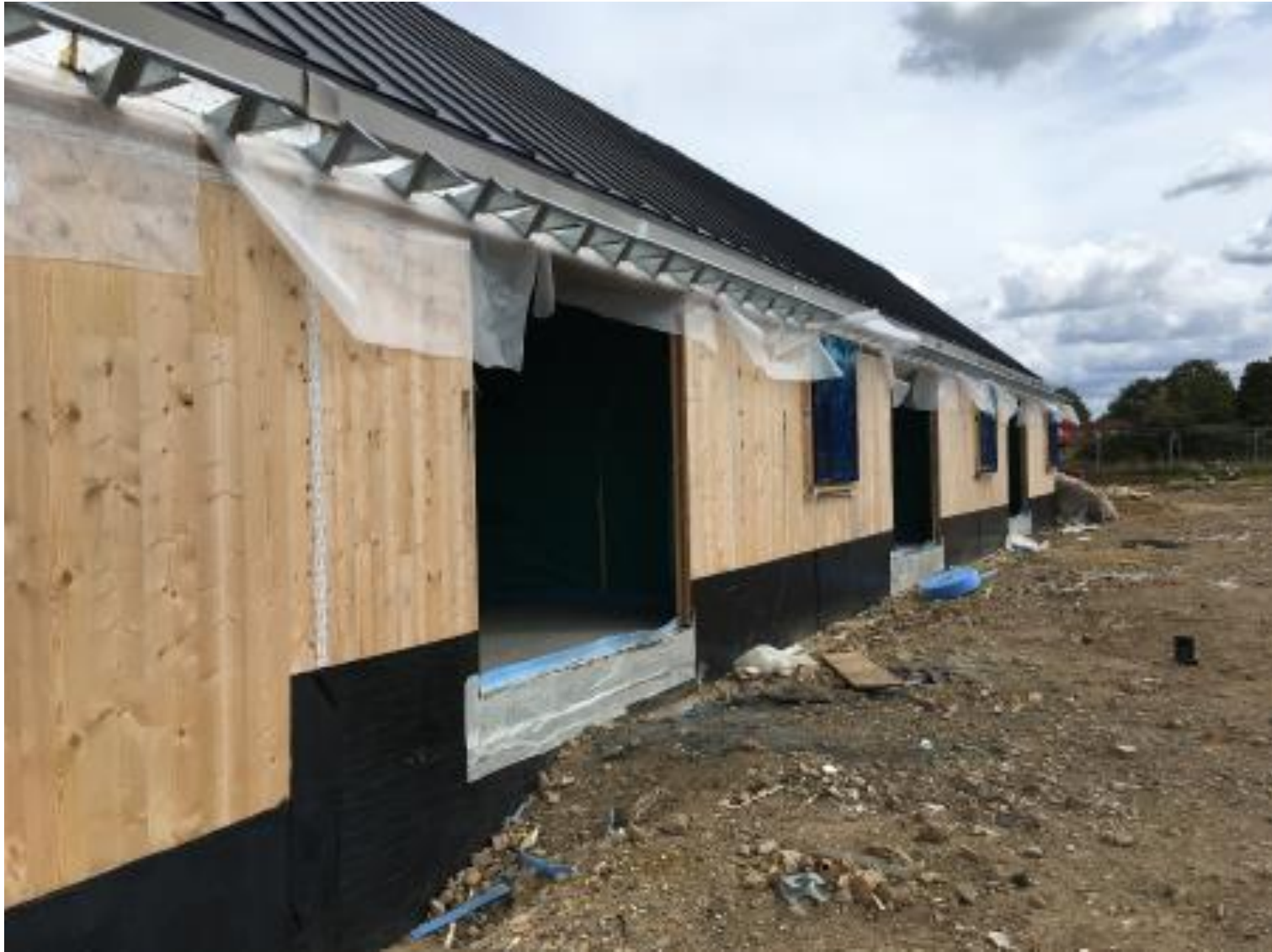
Photo 6 : View of part of Block B facing east
