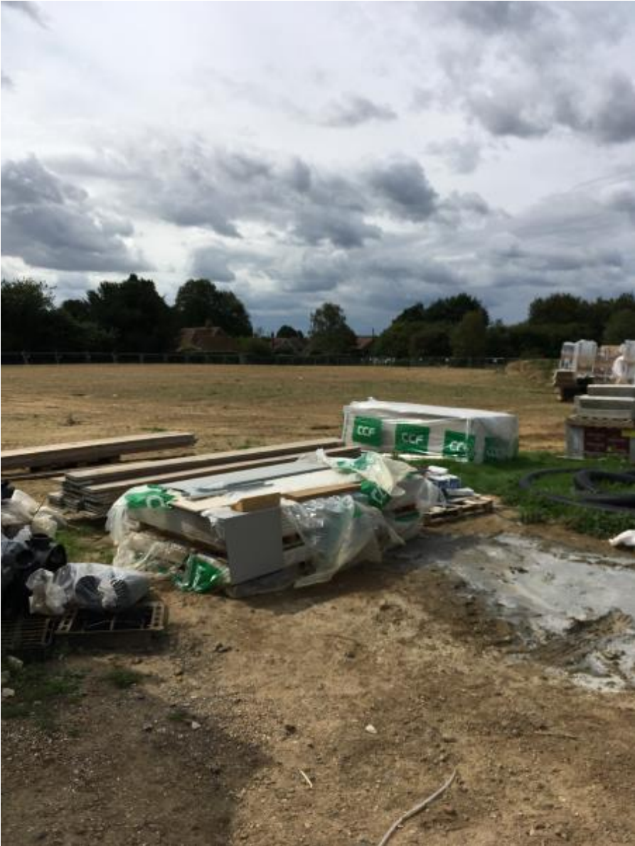
Photo 8 : View of open field facing south
