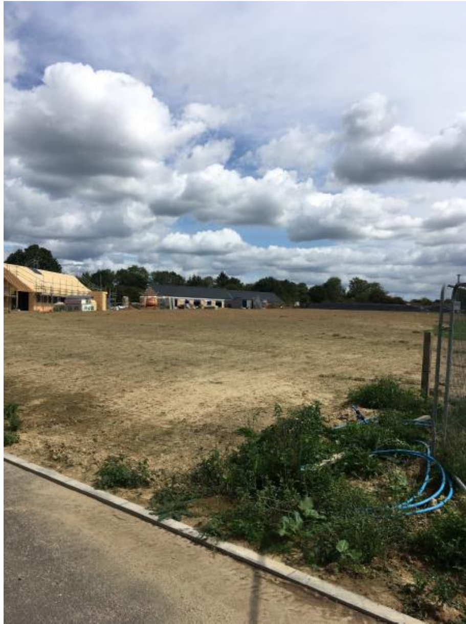
Photo 4 :View of Block D and Block B facing East
